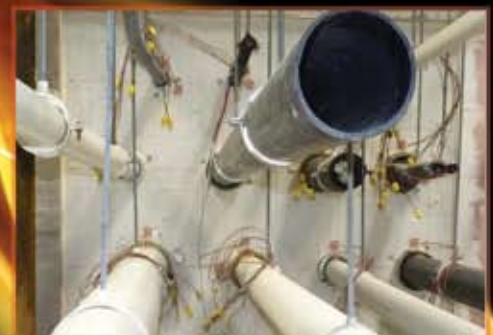
Non Fireside Prior to the start of one of our Fire Tests
