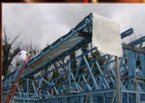
Starting Roof Wrap
