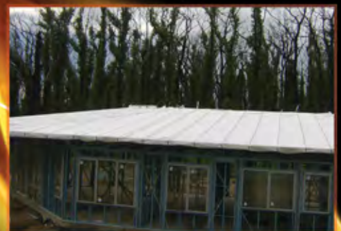
Completed Roof Sark
